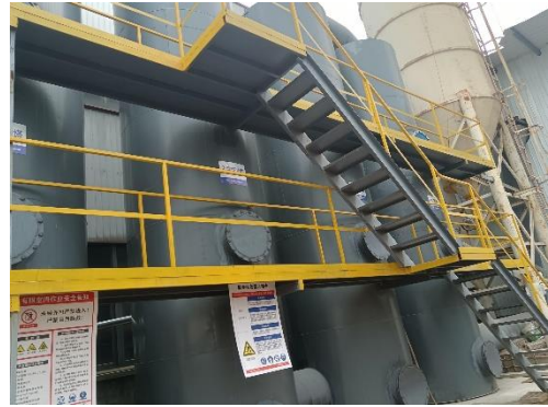
3级喷淋+电捕集除雾
