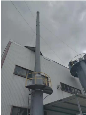
3级喷淋+电捕集除雾烟囱
